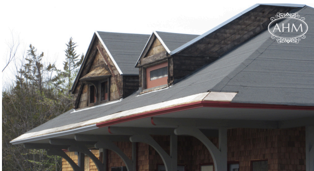
Photo of remodeled station in progress. The light-colored wood on the track-side eaves is part of the remodeling efforts, filling in the section that had been previously cut off.
