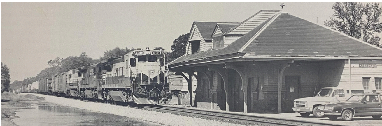
This 1967 Photograph shows how the eaves of the Station were cut to accommodate the growing size of trains.
